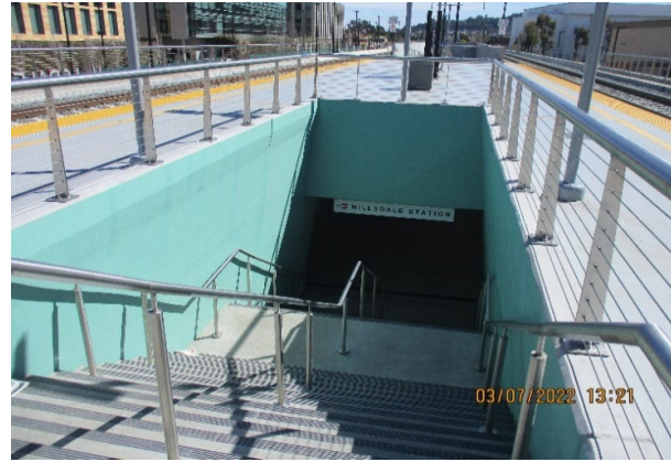
Photo 4 - Stairs Paint Touchup at Hillsdale Station
