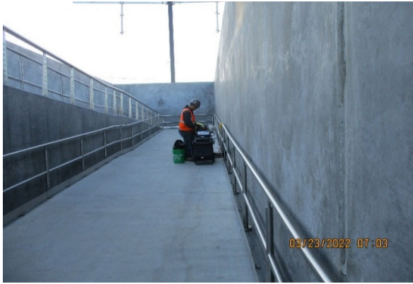
Photo 3 - South Ramp fixing plate kickers
