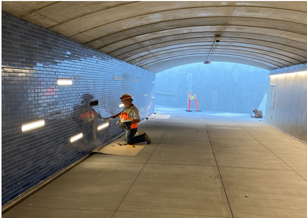
Photo 3 - Ped Underpass looking east
